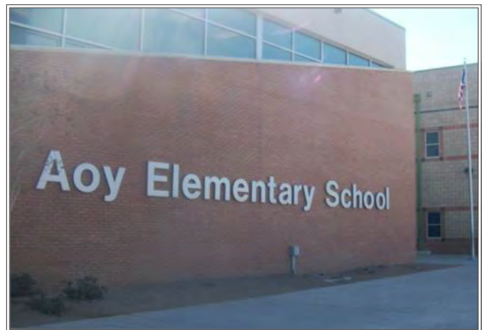
Aoy Elementary School features a more compact design than the conventional prototypes, allowing it to be sited in an established neighborhood.
