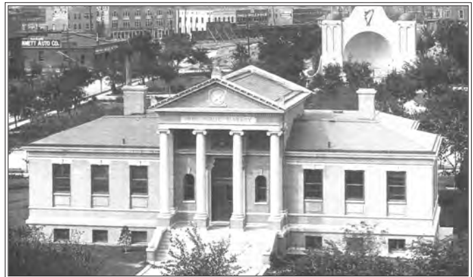
Original Carnegie library, opened in 1904 and demolished in 1968 (with Cleveland Square bandstand in background)
