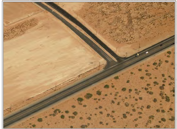
Zaragoza Road Existing Conditions
