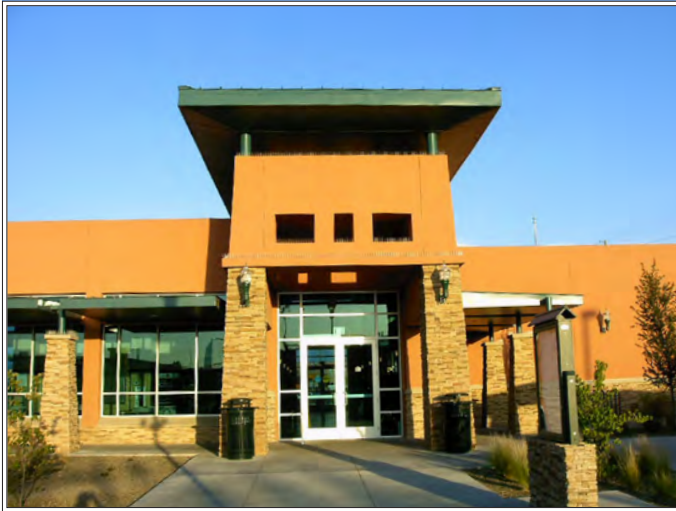
Downtown Transfer Center
