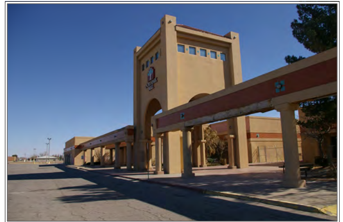
The Northgate Mall complex is currently vacant and unused and scheduled for demolition.
