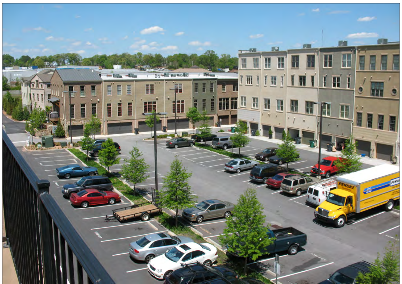
A mid-block parking court allows the street frontages to be free of garage doors and curb cuts, increasing pedestrian comfort and safety. Bioswales treat run-off with native plants and trees. Multiple windows and balconies increase natural surveillance. Glenwood Park, Atlanta, GA .
