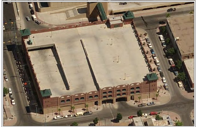
The Union Plaza Transit Terminal garage is an asset to the Union Plaza District because it provides plentiful parking. However its blank ground level façades have a dampening effect on other street activity.
