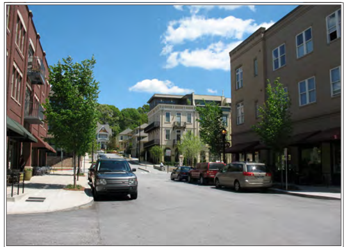
On-street parking. Glenwood Park, Atlanta, GA
