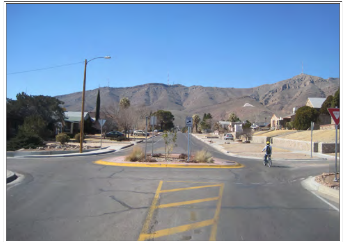
Traffic calming measures such as this traffic circle in Manhattan Heights can help create neighborhood Bicycle Boulevards.
