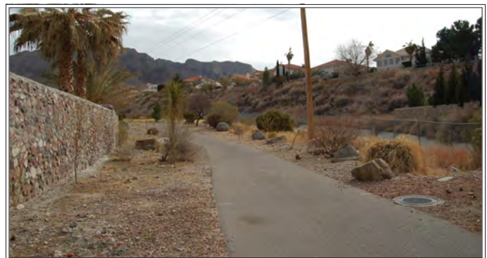
City of El Paso Trail System
