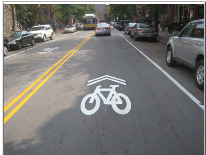
Shared use markings (sharrow)
