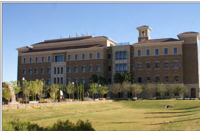
Grand public lawns of sod are used effectively when they also serve as drainage facilities such as at the UTEP Biosciences Research Building.
