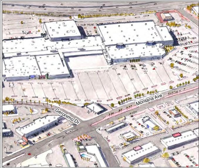
Existing Conditions: Bassett Place Mall is visible from I-10. The enclosed mall is surrounded by acres of parking. Parcels along Montana Avenue are developed in an auto-oriented manner.
