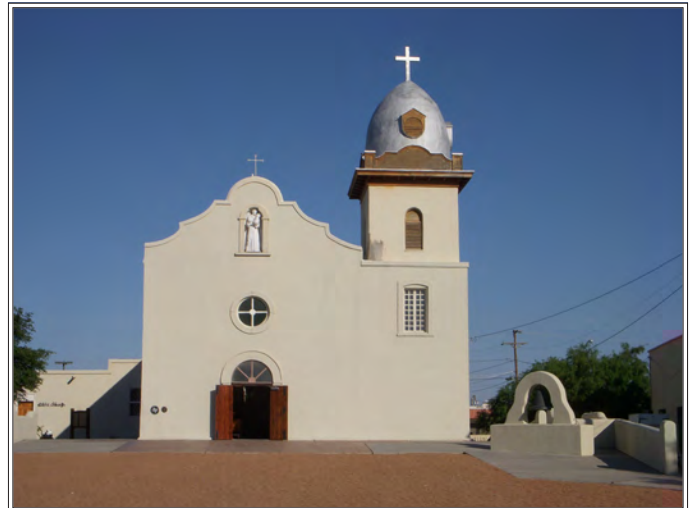
The Ysleta Mission is both a center of the Ysleta community and a landmark destination for visitors to El Paso. New homes, businesses, and services designed in context with the area, and with the pedestrian in mind, can enhance the experience of living in and visiting Ysleta.
