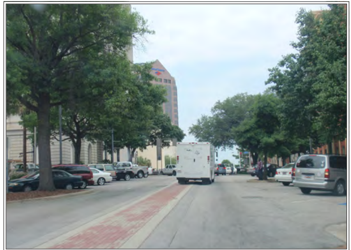
Safety Strip on Main Street, Columbia, SC
