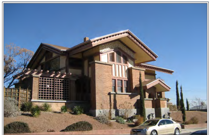
Henry C. Trost's largest concentration of buildings anywhere in the country can be found in El Paso. Trost & Trost architects was a firm of national repute at the turn of the 20 th century.
