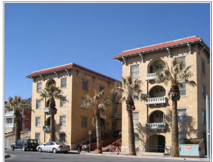
Apartment houses allow a great number of residents to live within walking distance of retail, services, transit, and public spaces. Well-designed multi-family buildings can offer both compact and spacious dwelling units.
