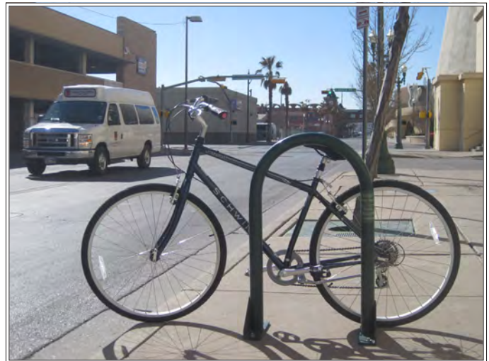
If used as intended, the improper installation of this U-rack bicycle rack places the bicycle within the vehicular right-of-way.
